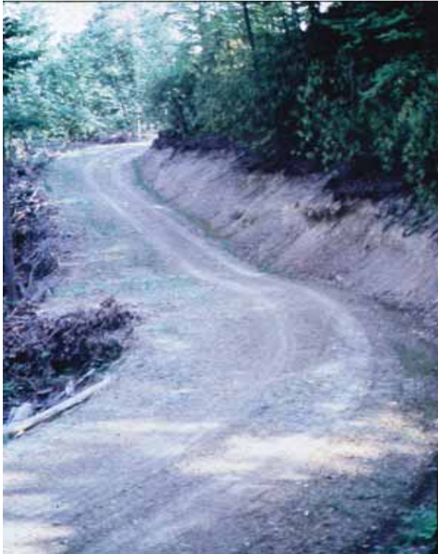
Photo 6.5 Broad-based Dip (Photo Source: Ohio State University Bulletin No 196)
