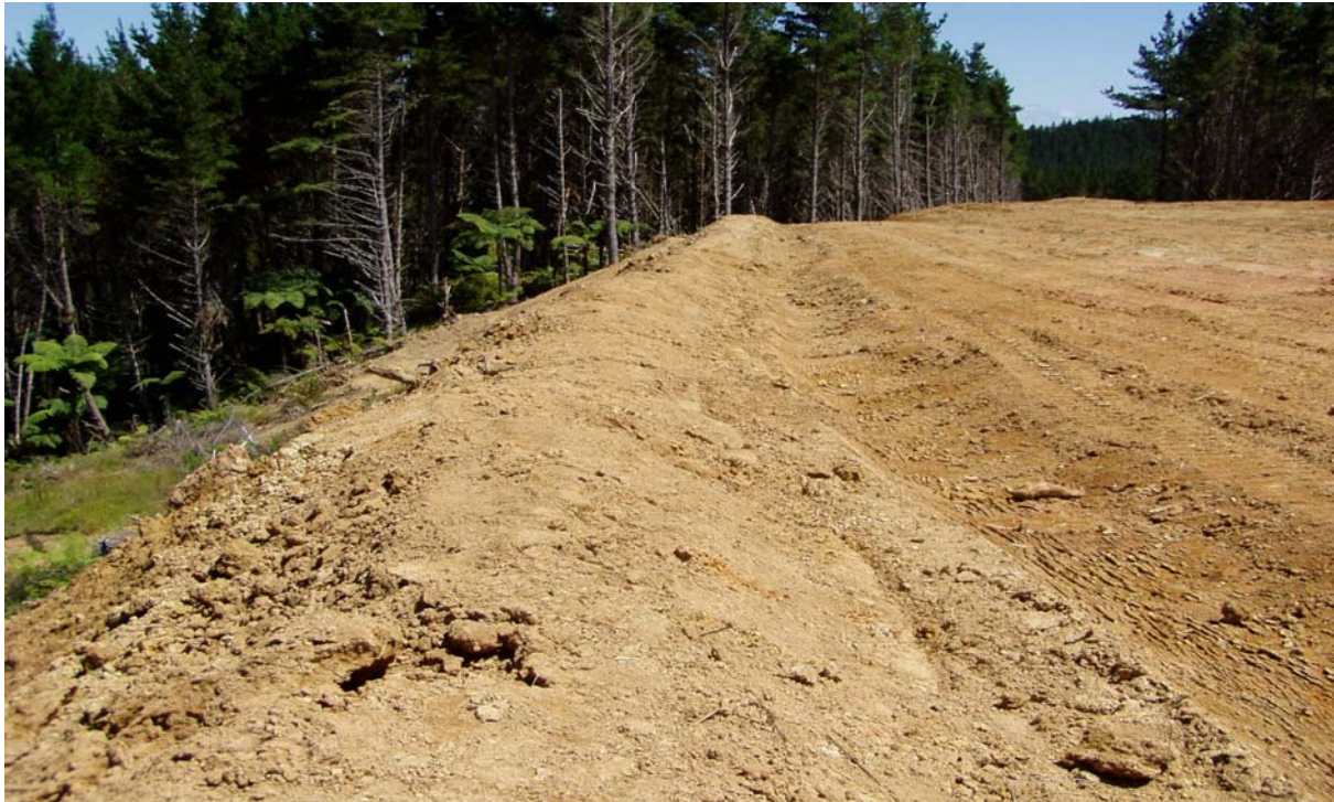
Photo 6.2 Diversion Bund installed on edge of landing site to direct water flows into a sediment control
