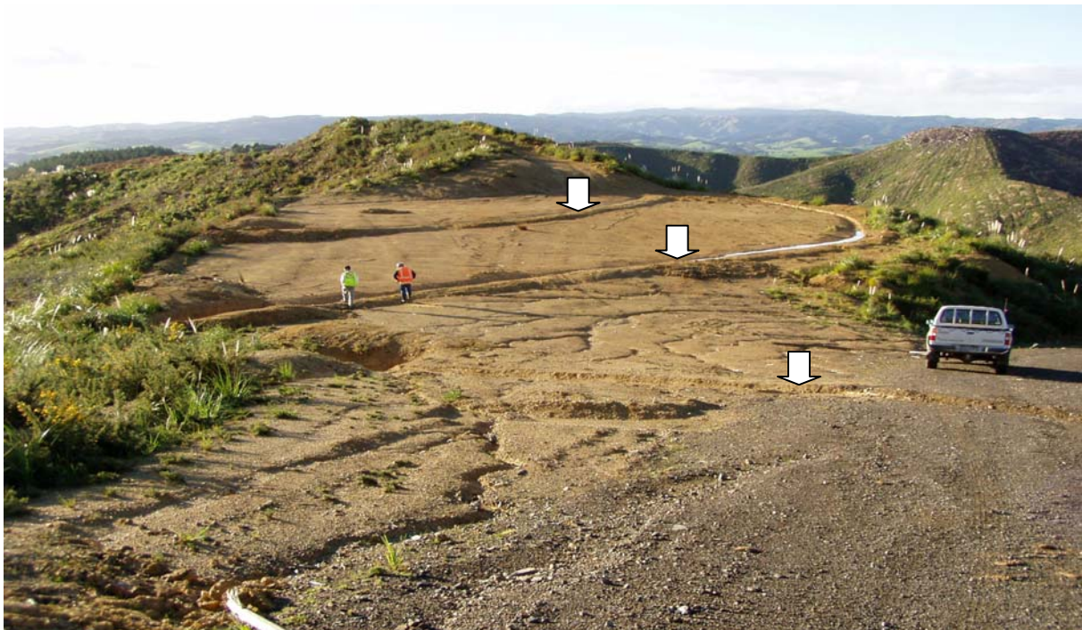
Photo 6.4 Cutoffs in road and landing site (arrows indicate the position of the cutoffs)
